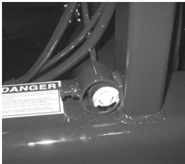
Figure 6. Remote shut down receptacle
