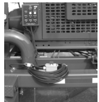
Figure 8. Remote shut down pendant
