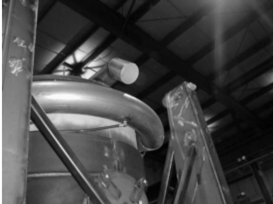
Filter Fig. 2 Bag house with hopper connection hose removed.
