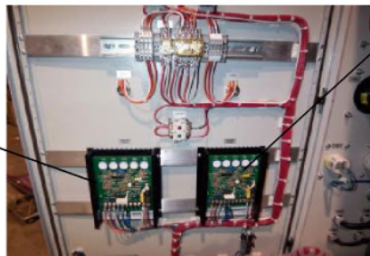
DC Drive For Fixture Drive Motor
